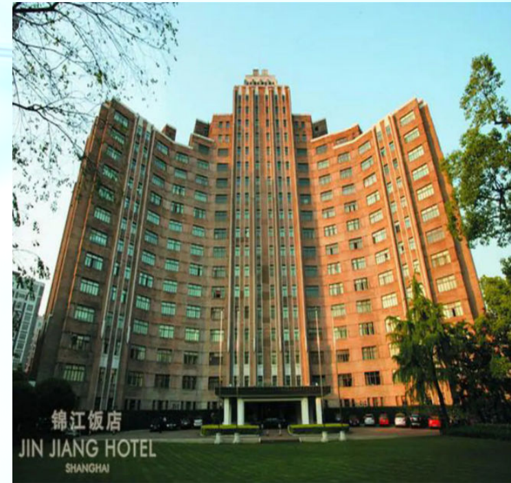
320,000 – GPD Bio-Pure (ACT) System constructed in the basement of the Jin Jiang Hotel and Commercial Center in Shanghai, China
